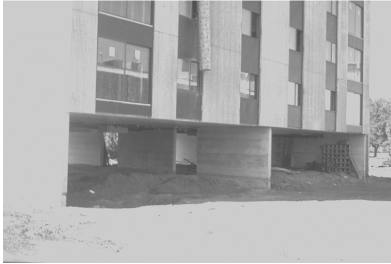
Figure 5-9: Building elevated on parallel stem walls.
