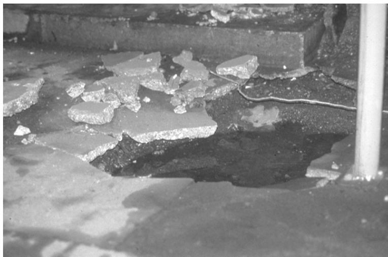
Figure 1-19. This basement floor broke from hydrostatic pressure
