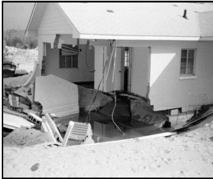
Figure 1-16. Beaches are particularly susceptible to undermining of foundations due to velocity flows.
